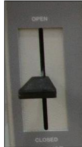
Figure 6. Damper Positions.
