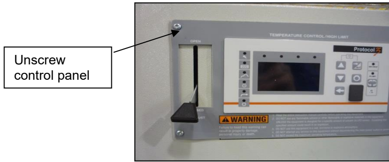
Figure 11. Control panel removal.
