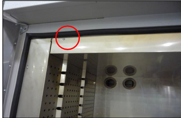
Figure 20. Remove Screws to Remove Ceiling Plate.
